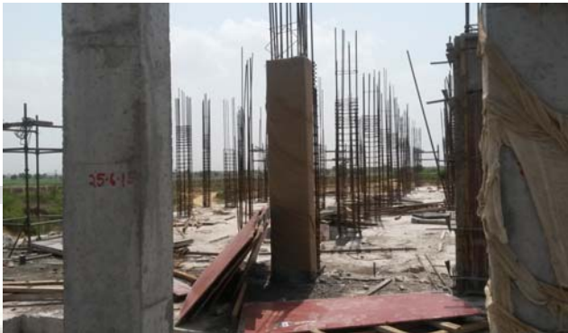
Column works for the second roof level of Guest House
