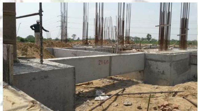
Tie Beam works in progress for SNSS Building
