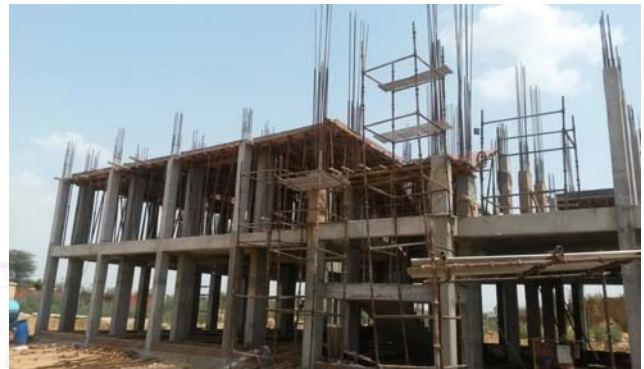
Under construction Block of Guest House
