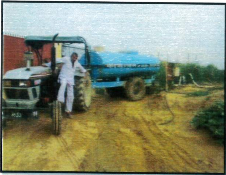
Water Sprinkling at Site.
