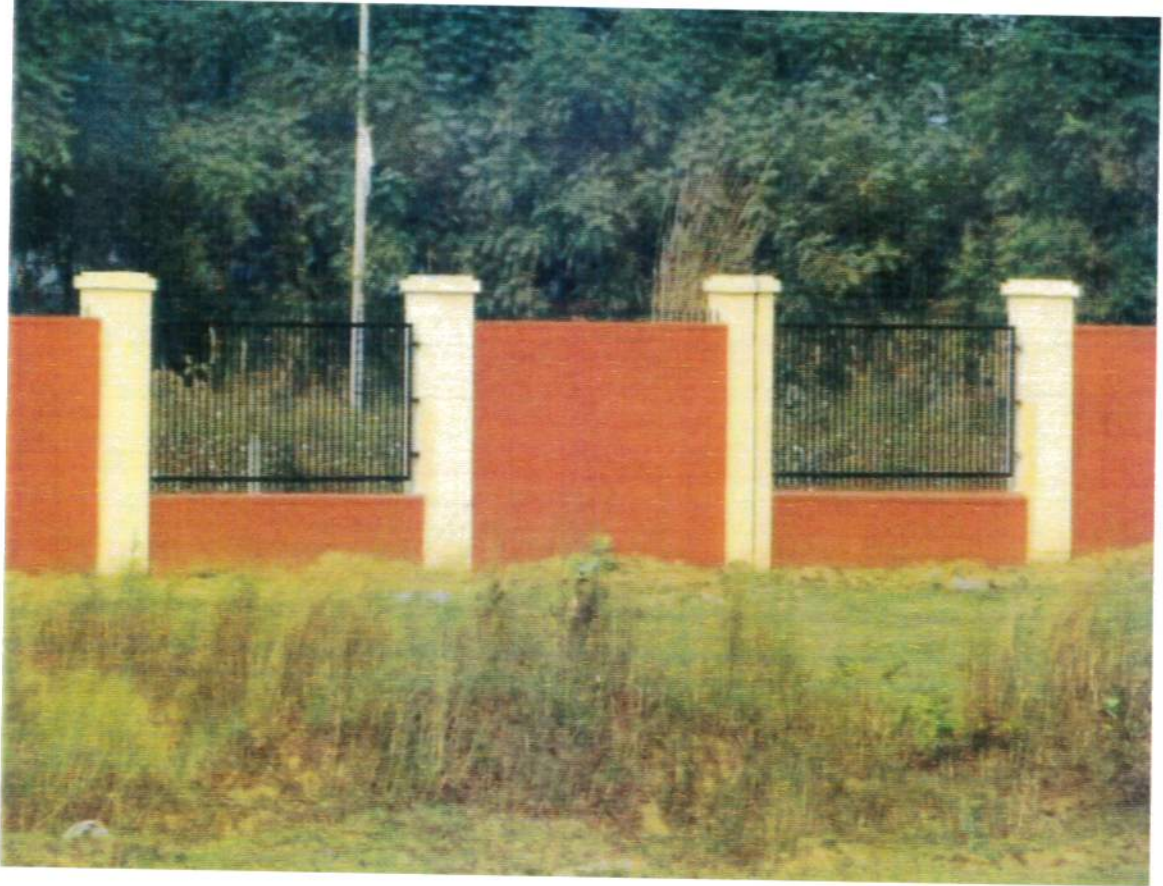
Site Barricade with High wall
