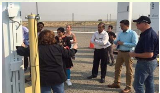
Indian delegates visiting Radiation Monitor Portal test station installation
