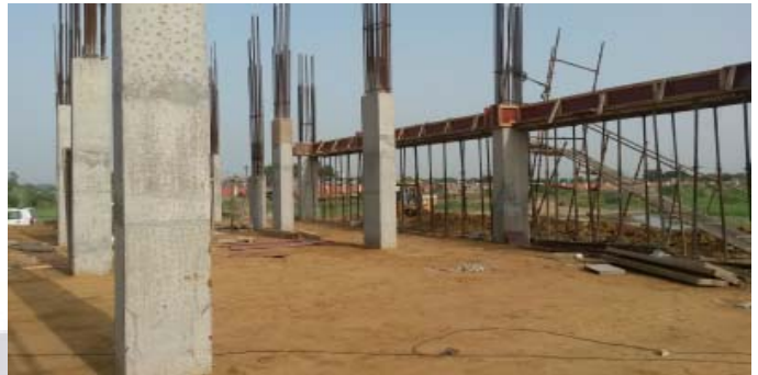
Column raising in progress for SNSS Building
