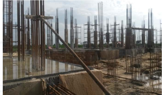
Column raising in progress for SNSS building
