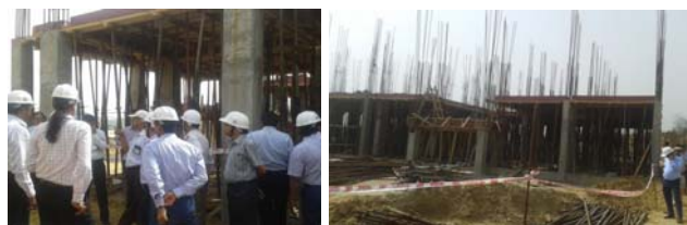
Ongoing works for Block-A of Guest House
